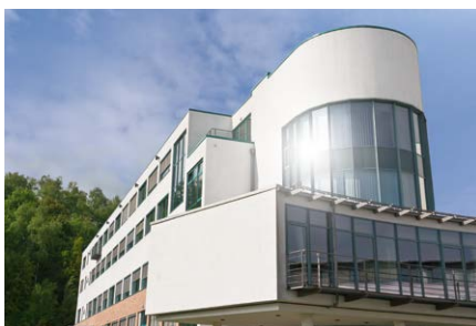
Headquarters in Dresden, Germany
